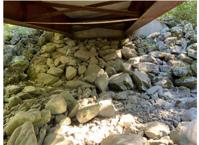
Left Bank Abutment when facing downstream
