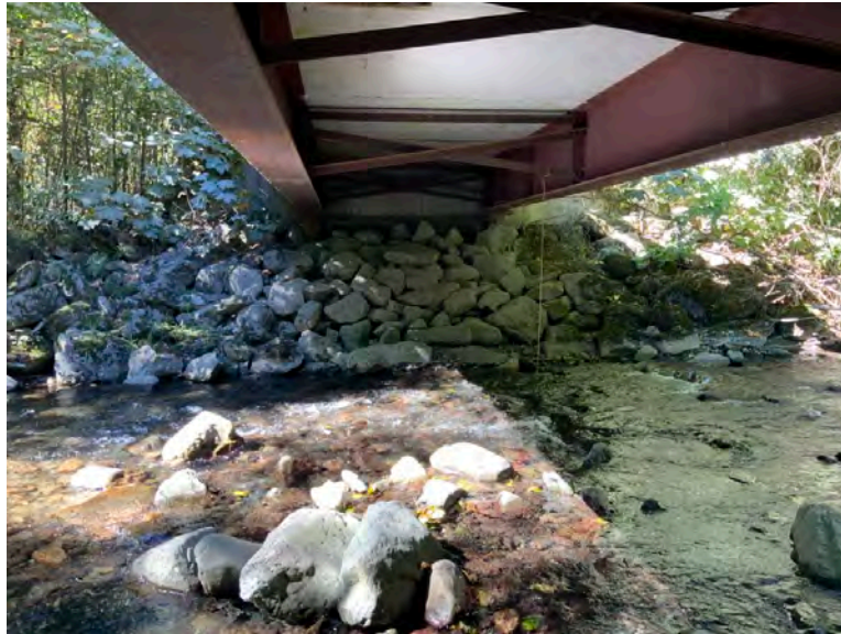
Right Bank Abutment when facing downstream
